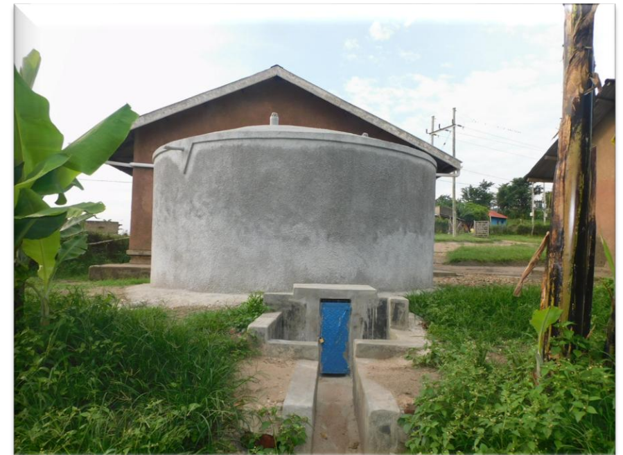
30,000L Rain-water Harvesting Tank at Katokye P/S
