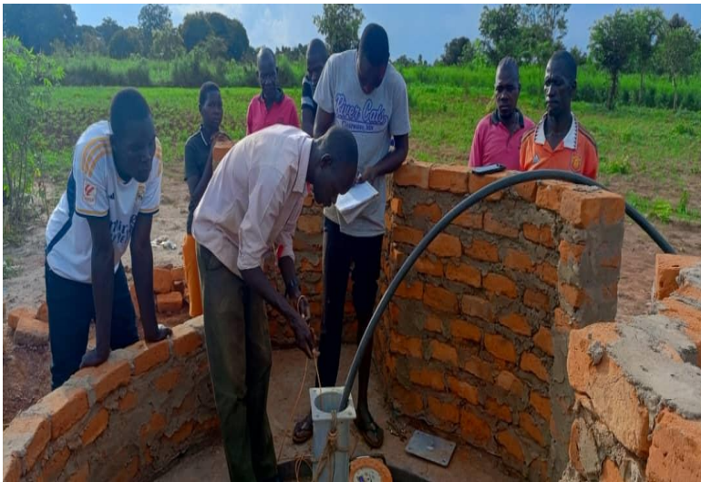
Acanwing pump testing on going
