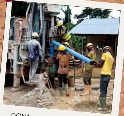
DONA encasing a deep well in Ghana after accessing water.
